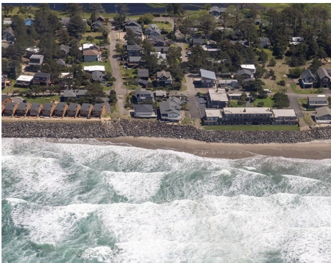
Left: Extensive riprap placed on the beach in Neskowin, OR, make stretches of beach impassible. (📷 Rena Olson) Right: Public beach access points are closed off due to failed riprap and rock armoring.
