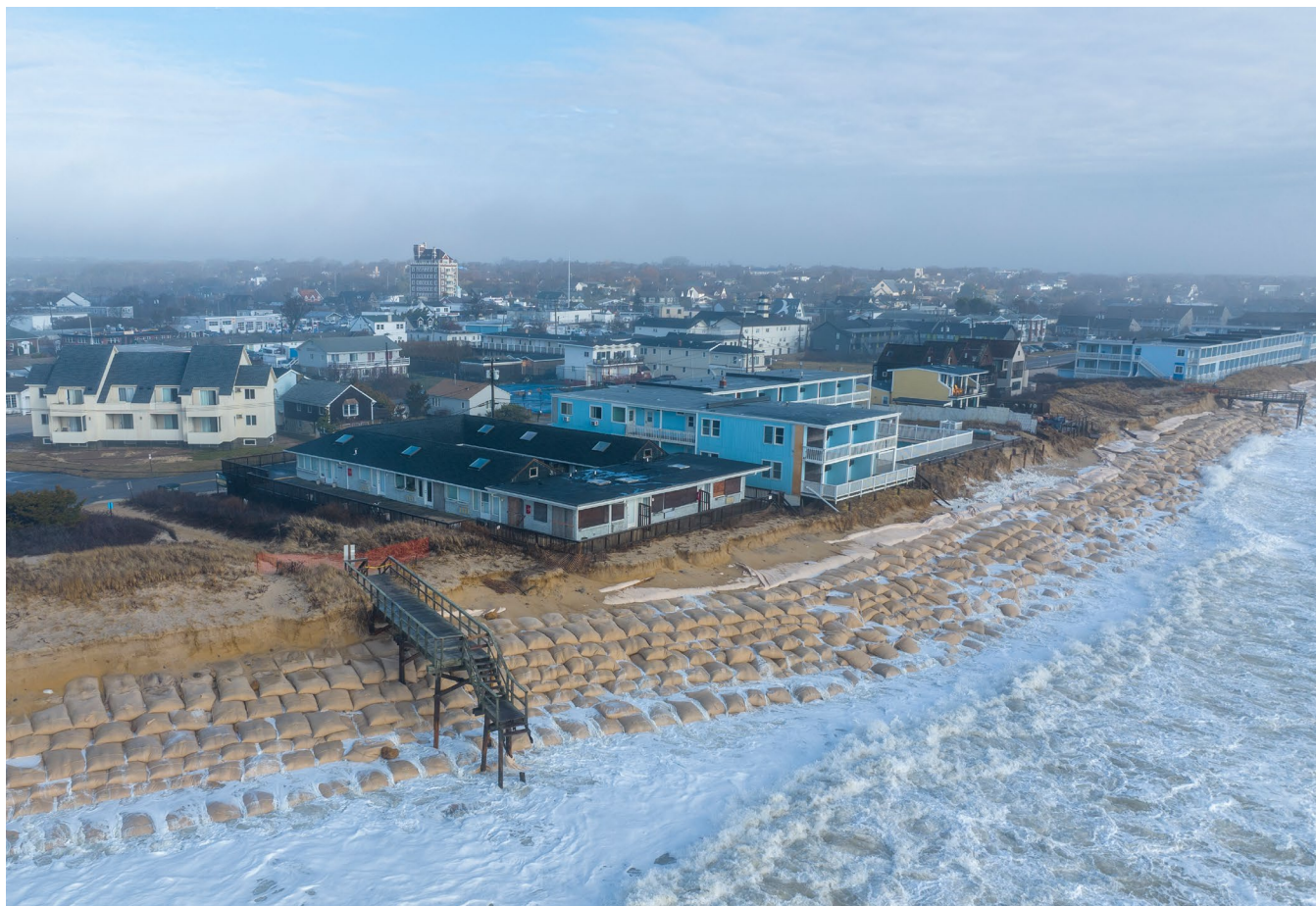
Extreme weather threatens properties along the coast of Montauk, NY, demonstrating the negative effects of using short-term armoring as a long-term solution. (© James Katsipis)
